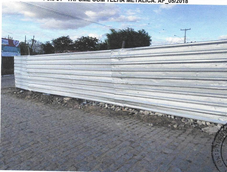
Foto 02 – TAPUME COM TELHA METÁLICA. AF\_05/2018
