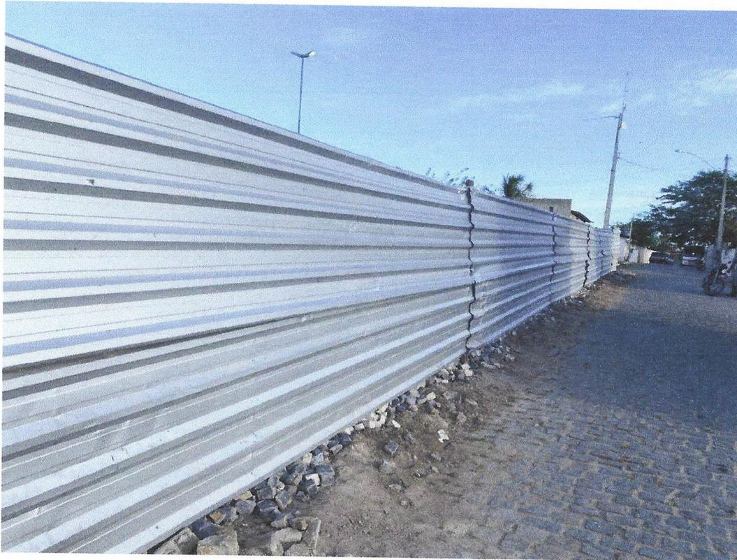
Foto 03- TAPUME COM TELHA METÁLICA. AF\_05/2018
