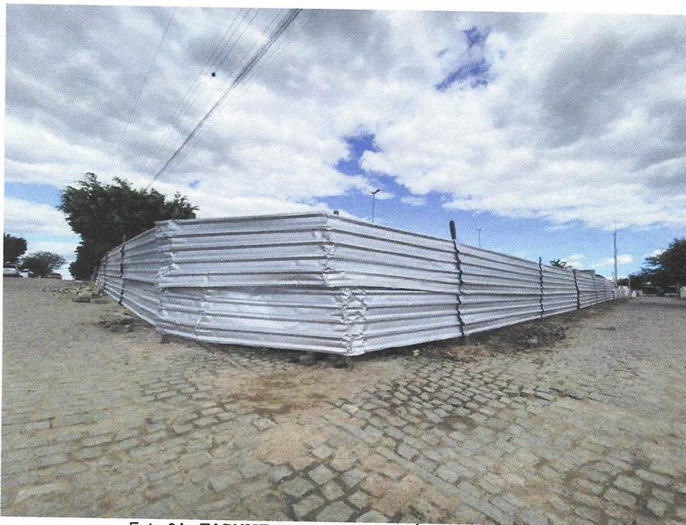
Foto 01 - TAPUME COM TELHA METÁLICA. AF\_05/2018
